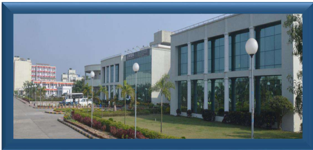
Management Development Institute, Murshidabad – Campus
